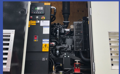
Electricity is provided by a powerful diesel generator as well as shore power if desired.
